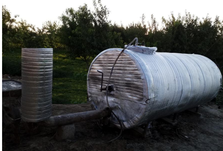
Figure-3. General view of a pilot production biogas plant
