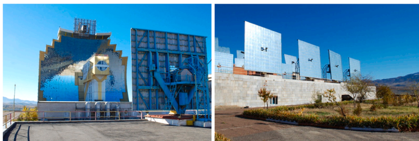
Fig. 2. Large Solar Furnace (LSF), Parkent, Uzbekistan: (a) segmented parabolic concentrator and focal tower; (b) heliostats field [43].
