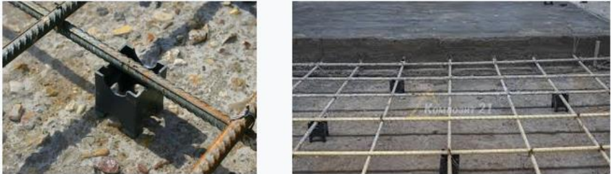
Figure 1 View and location of steel frames of the road reinforced concrete bridge protective layer
