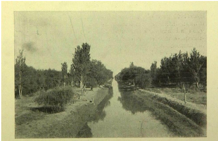
Fig. 1. General view of the channel of Emperor Nicholas I
