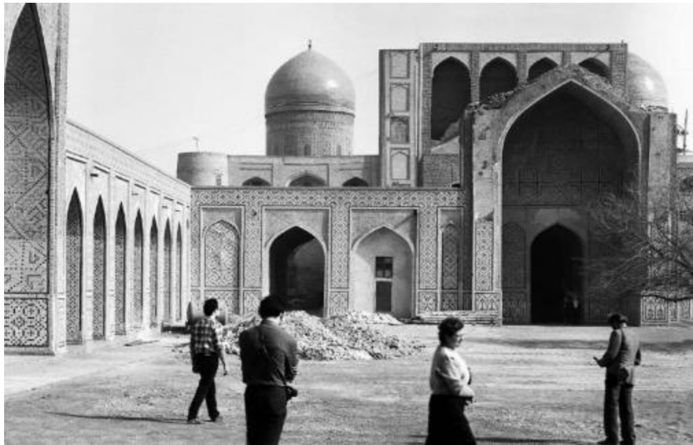
Mosque Kalyan. Courtyard. 1970
