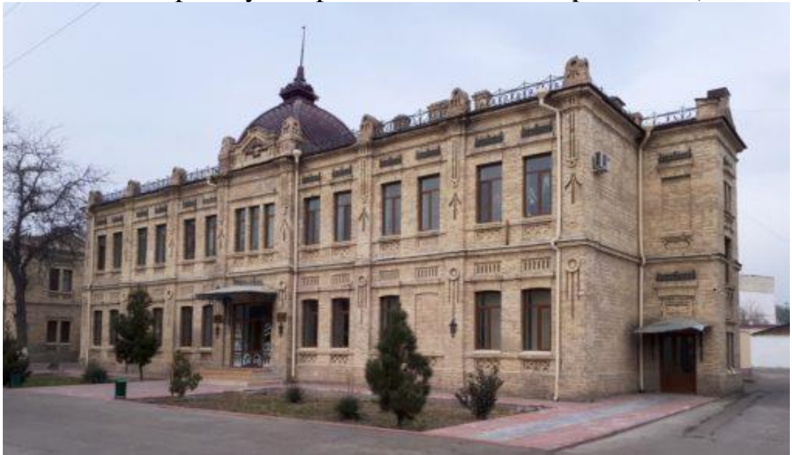
The building of the open telegraph office. 2018
