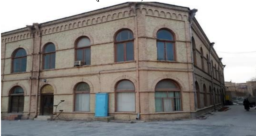
Savva Morozov Trading House. 2019
