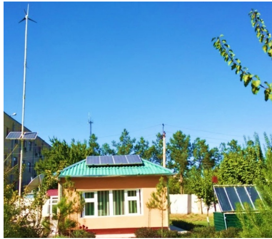
Fig. 1. General view of the experimental solar house (Karshi city).
