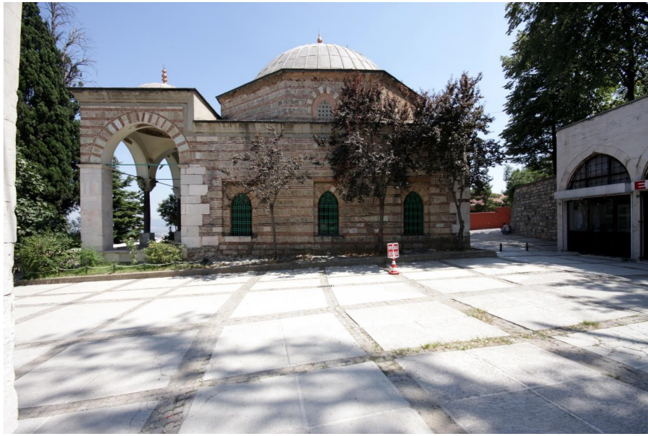
Figure 4. General View of the Yıldırım Bayezid Mausoleum in Bursa.
